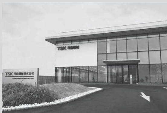
図2 事務所棟正面 Fig.2 Entrance of office building.
