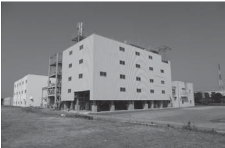
図5 相模川流域右岸処理場焼却設備の外観写真① Fig.5 The picture of Sagami River basin right bank treatment plant incineration system(1)
