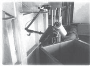
図12 ④しき脱水機用ホッパーの監視 Fig.12 Monitoring for the hopper of debris dewatering machine
