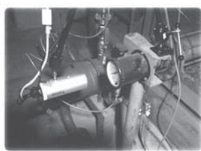
図10 ⑦ケーキ圧送PGの監視 Fig.10 Monitoring for the pressure gauge of cake pump
