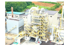
Waste treatment facility
