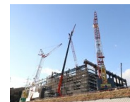
Waste incinerator furnace plant construction
