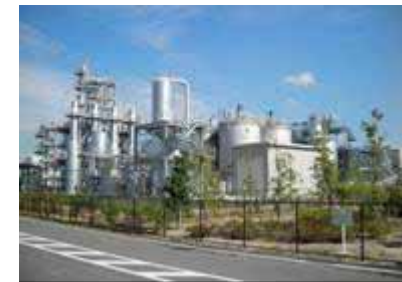
Biomass ethanol manufacturing plant
