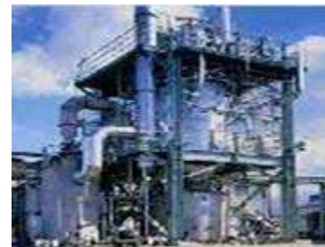
Waste liquid combustion facility
