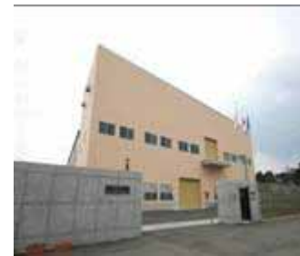
Samukawa Water Services building (PFI operations: consolidated from March 07 period onwards)
